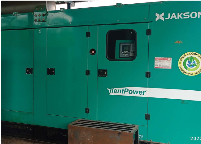
CUMMINS make -Diesel generator Set, capacity of 380KVA - Stand by Power Source for emergency operations.
