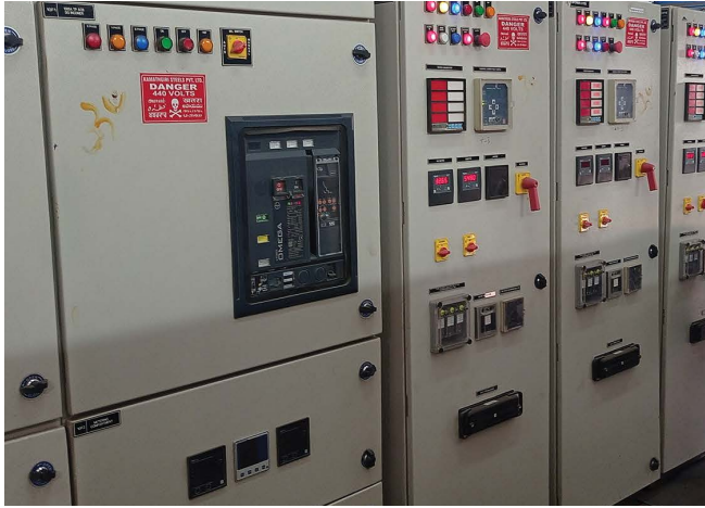
L.T.- Power Control Station with distribution Panel Boards with Capacitor banksfor total Machinery and equipment of the Plant
