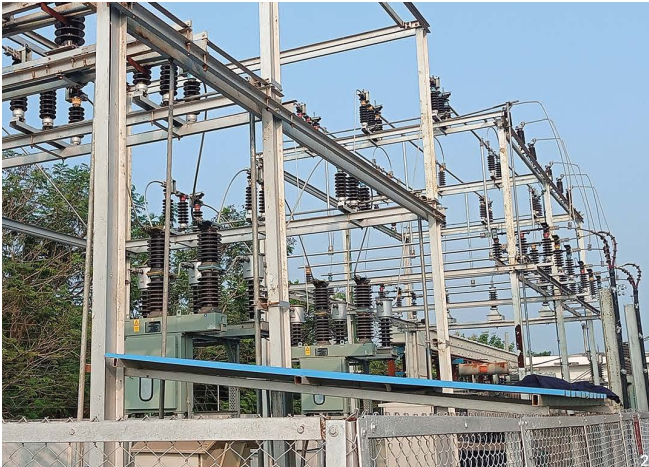
High Tension Powered Sub station with VCB - AB switches- 2.5MVA Transformers(3nos) Assembly
