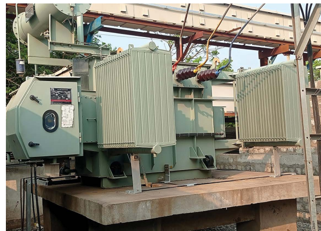
Step down 2500KVA, HT Transformers assemblies with 33KV/415V potentiality
